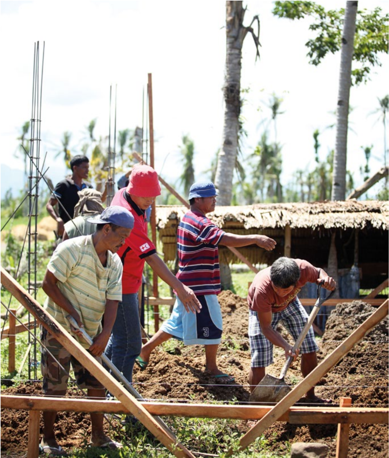
Tropical cyclone shelter construction, the Philippines.
